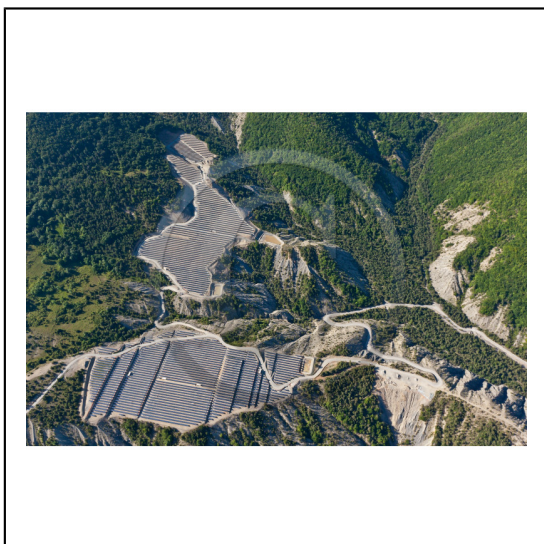
Alpes de Haute-Provence, 04, Village de Curbans, construction par GDF-Suez, sur 300 hectares au Col de Blaux, de la plus grande centrale solaire photovoltaïque d'Europe. // Alpes de Haute Provence, 04, Village of Curbans, construction by GDF-Suez, on 300 hectares on the Col Blaux, for the largest photovoltaic solar power facility in France (south east of France)...
